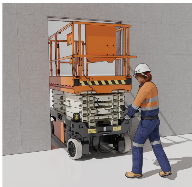
Figure 25 – Operator 'walking' the EWP through restricted area, using the removable control
