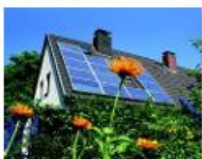
Panels parallel with plane of roof- Exempt
