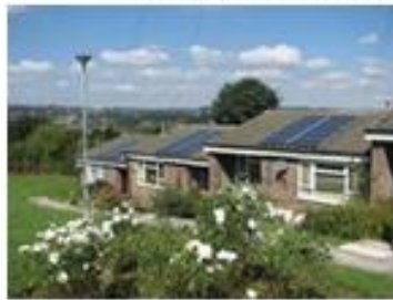
Different roof planes and independent roof structures.
