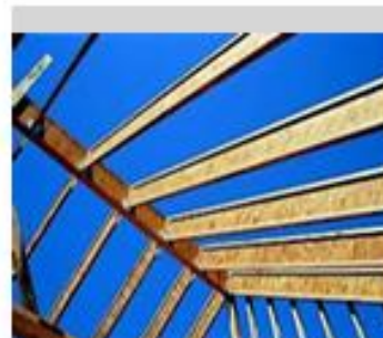
Different planes. Not independent roof structures.
